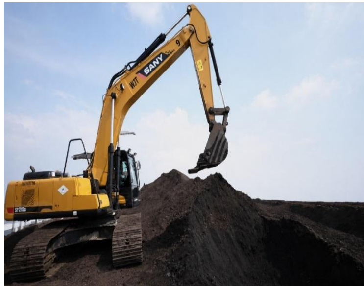
Gambar 4. Excavator SANY SY215C
